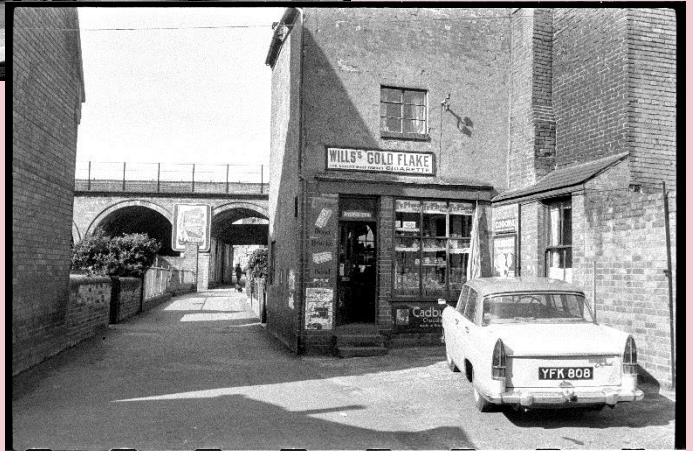
Photos are of Carden Street Clearance Area, 1959; Infirmery walk, late 1950s; the Public Hall, Cornmarket, demolished in the 1960s
